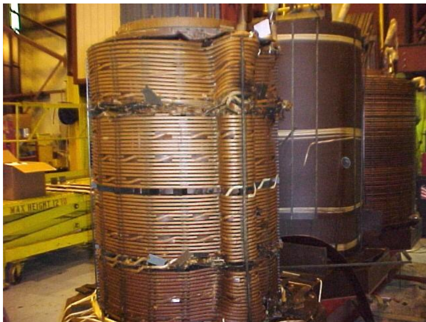
FIG 13. Collapsed winding photograph and loose connections in the previous test transformer.
