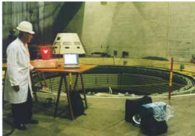
Fig. 1. EDA test in Iberdrola's hydro power plant.
